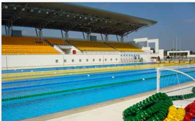
A typical 50 metre Olympic Pool.
