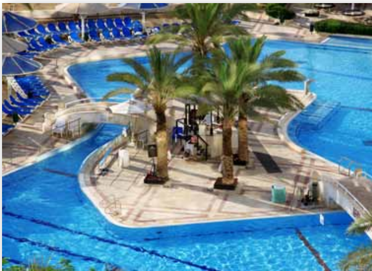
Odd shaped pools should be sectioned off into basic shapes for determining water volumes.
