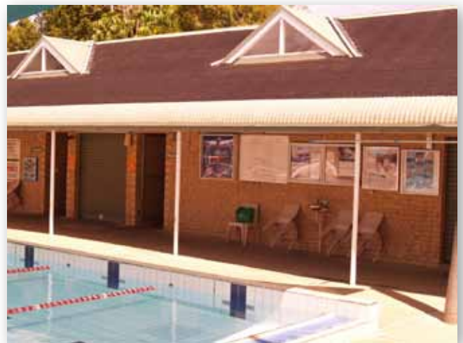
Solar panels installed on the roof of an amenities block.
