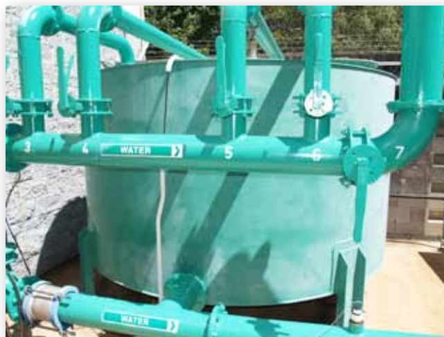
An efficient sand filter system is easy to manage.
