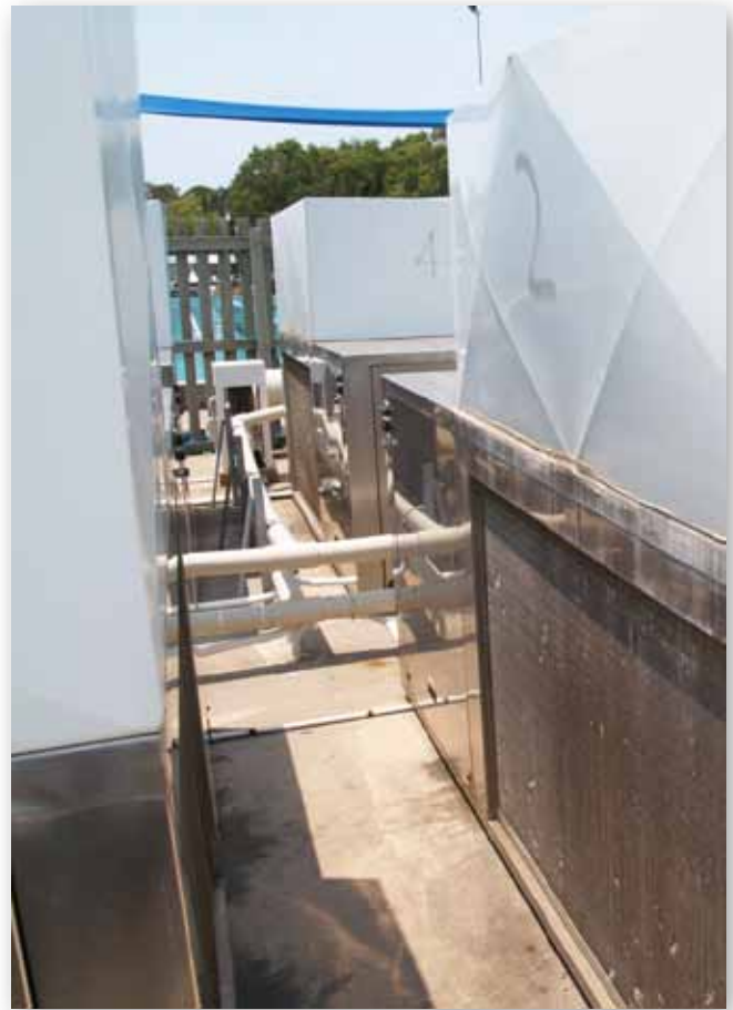
Electric heat pumps provide a great source for heating swimming pool water.
