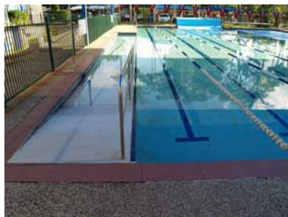
Ramp entry to main pool.
