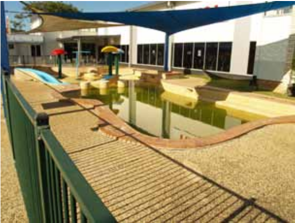
Pool concourse in satisfactory condition.
