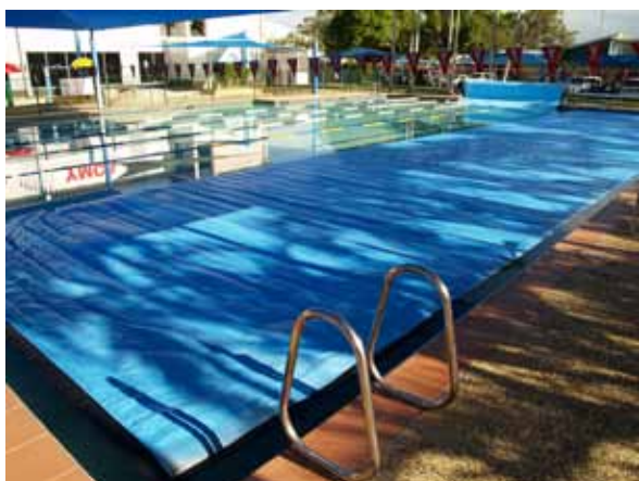
Depth markings to be upgraded.
