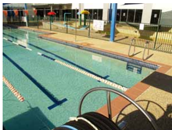
Depth markings to be upgraded.
