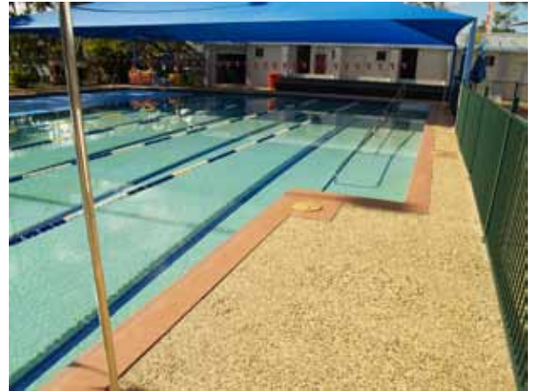
Pool concourse in satisfactory condition.
