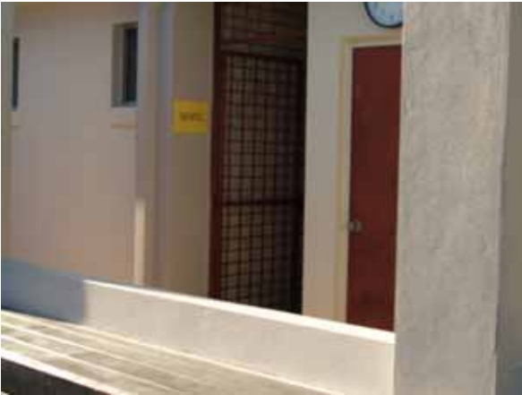
Upgrade amenities signs.
