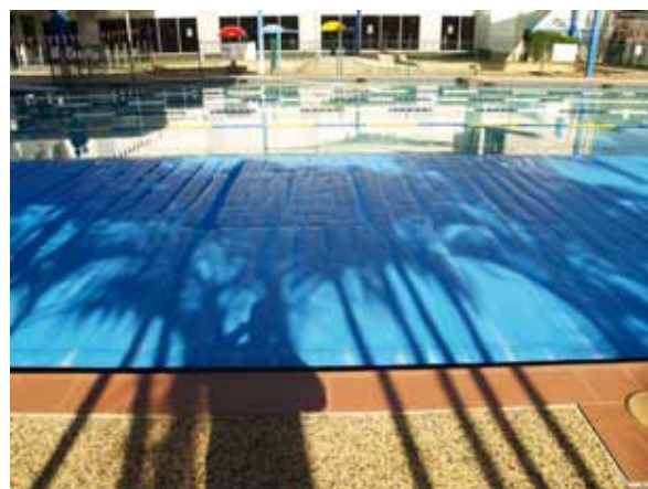
Depth markings to be upgraded.
