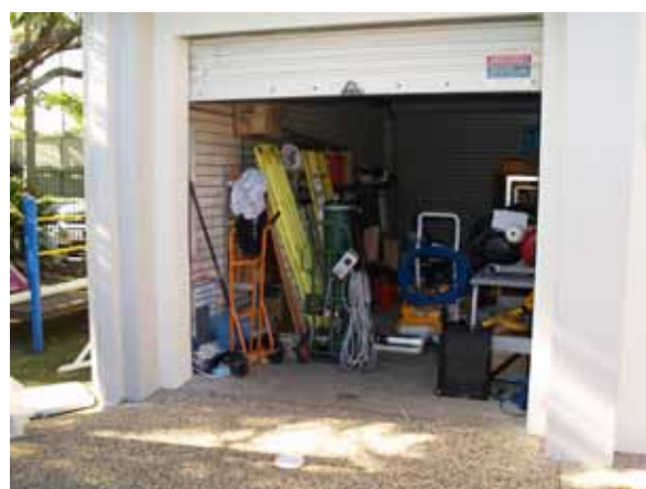
Storage area to be converted to first aid room.
