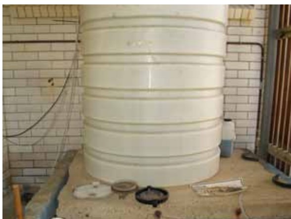
Bund to be replaced.
